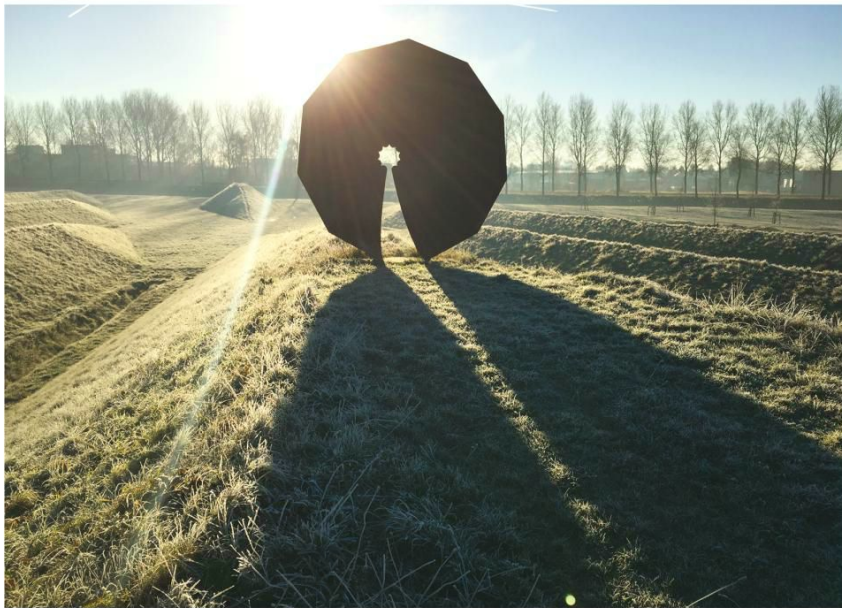
LEFT Noise-dampening earthworks from H+N+S and a sculptural touch at Buitenschot.
